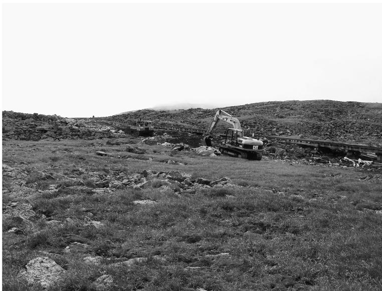
Figure 1. A backhoe was used in the summer of 2008 to dig a trench on Mount Washington, just north of the Cog Railway, to bury an electric cable and a fiber-optic line. The work severely disturbed the plant communities from the bottom of the mountain to the summit, through the alpine habitat, removing all plants and much of the organic soil. A survey was done to assess recovery of the alpine community four years later. (Photo by Kent McFarland)
